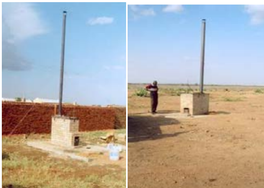
Figure 14.3 Double-chamber incinerator in a health-care centre dumping site
