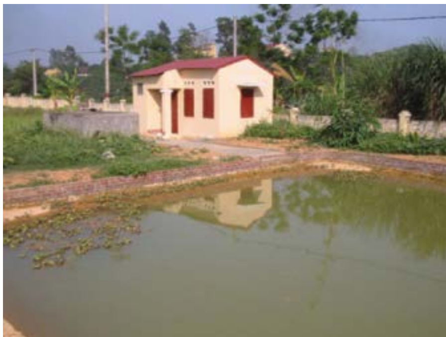
Figure 9.7 Basic lagoon system at a hospital
